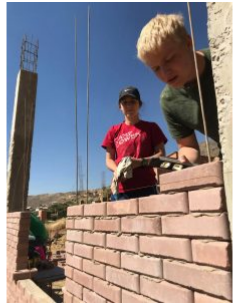
Getting that wall built!
